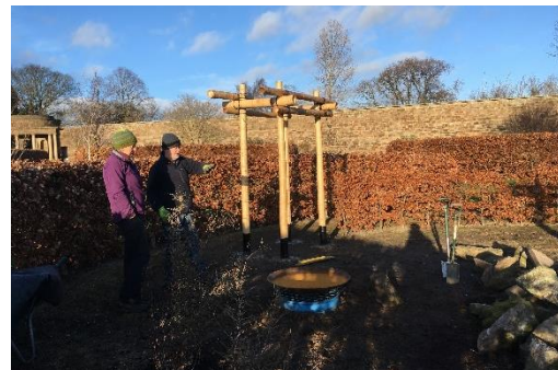
Sound garden under construction
